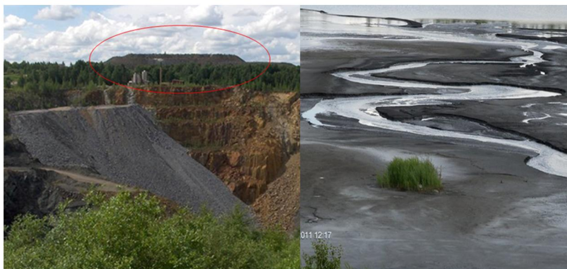
Fig. 1. The unavoidable mine waste includes waste rocks and mine tailings. Unless they are reused or recycled, they are stored as rock piles on the outskirts of the pit (left, marked with red) and as tailing basins (right). Photos: Hitura by S. Lavikko
