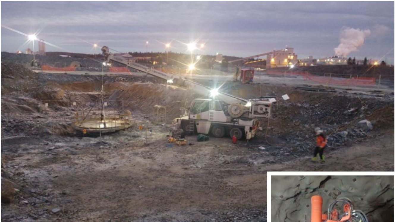
Temporary sinking platform with mill in background
