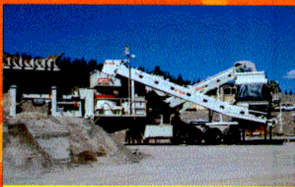
Holmlunds Schakt AB, Sweden – a mobile secondary aggregate production plant
