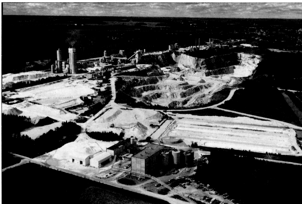
Partek Lappeenranta Works
