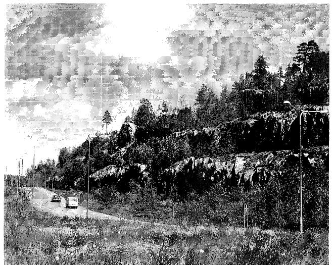
Fig. 2. The aggregate from this stepped rock at Vantaa was used as fill for the adjacent motorway and to some extent also as material for the base courses of motorway.
