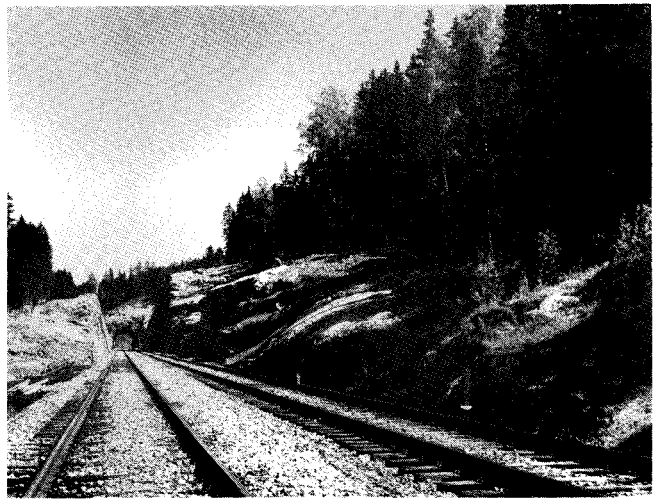
Fig. 1. Finnish rock presents a challenge to the designer and constructor, but is also a source of raw material. Espoo railway tunnel. The high-quality railway ballast was extracted from local rock.
