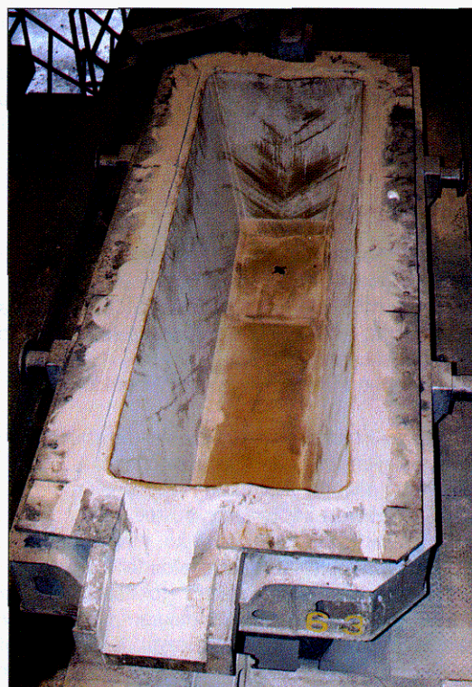
Fig. 3. The new tundish of Rautaruukki Steel, lined with 30 mm thick dry insulating cover mix that creates the bond also by the remaining heat of the backing lining. This method enables energy savings, effectivity, a possible reduction of hydrogen in the molten steel, as well as a possible reduction of the amount of circulating tundishes. (Photo by Mr Raimo Aho, Rautaruukki Steel).
