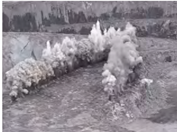
Fig. 4. Gas ejection in both the presplit holes close to the slope and the first row of production holes.
