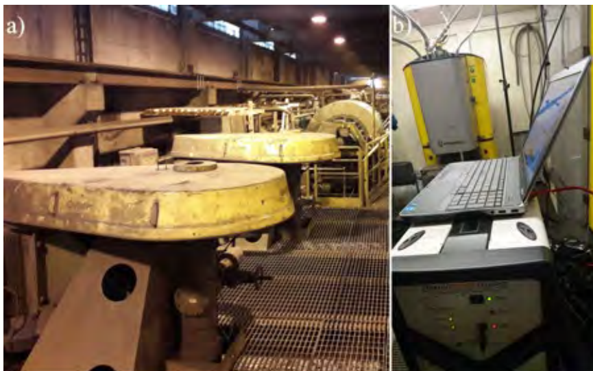
Figure 2. a) Pyhäsalmi beneficiation facility's froth flotation tanks, b) Raman instrument connected to online XRF analyser at Pyhäsalmi.
