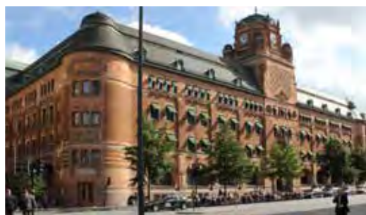
Old Central Post Office Building Vasagatan 28, Stockholm, Sweden
